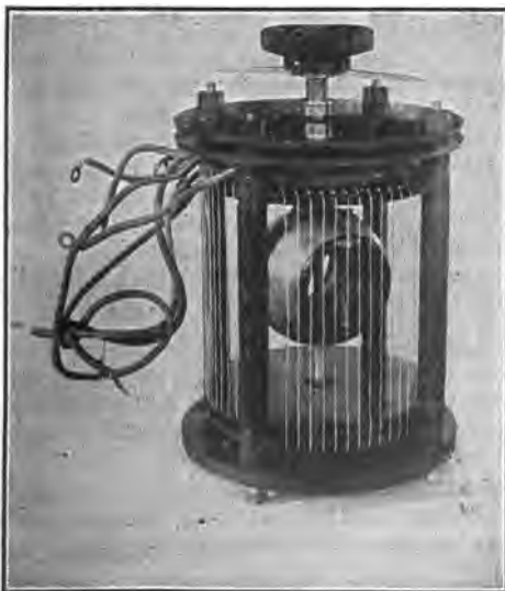
Fig. 272—Detail of the Radio Goniometer.
